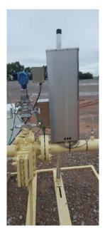
The photo demonstrates the interference with the manifold and the orifice fitting. Similarly, a composite sampler will not fit in the first pressure tap of a two-inch meter.
